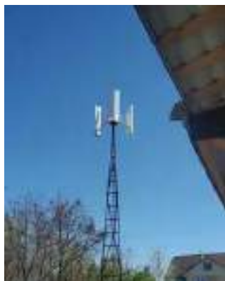
Fig. 6. Large domestic wind turbine
